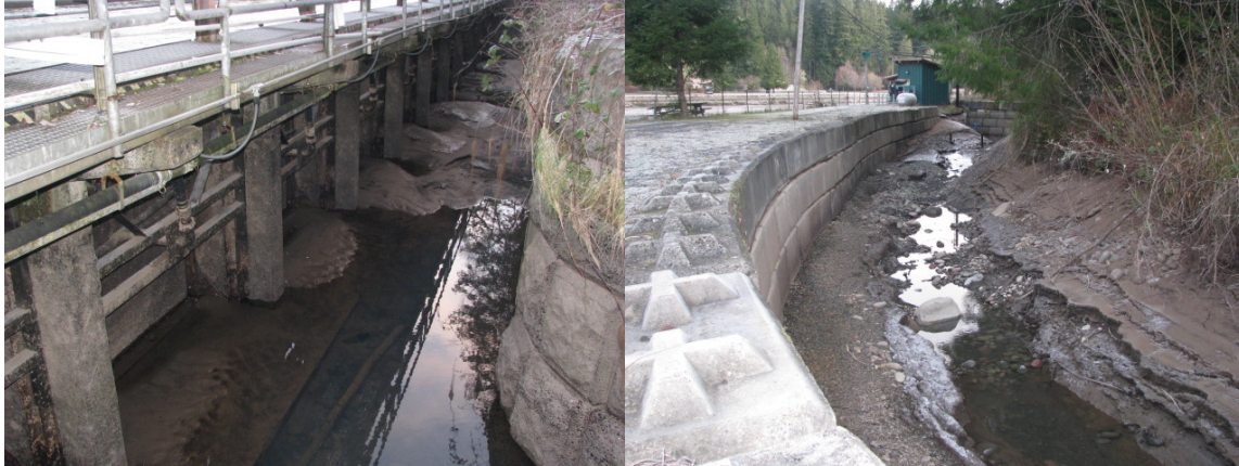
Behind Intake Screens
